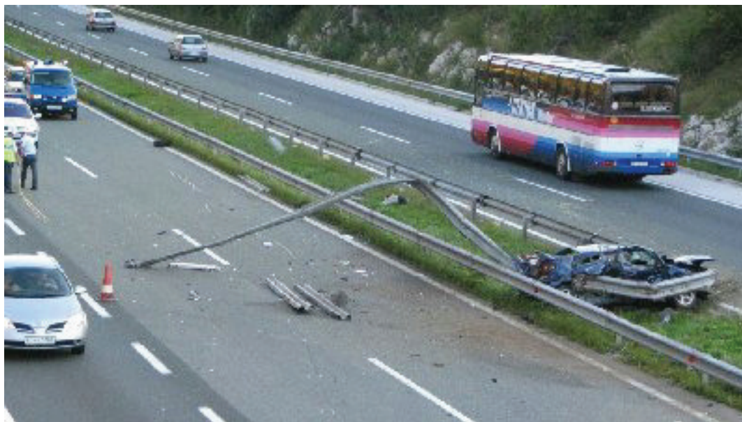
Picture No 2: Failure on Containment Level
